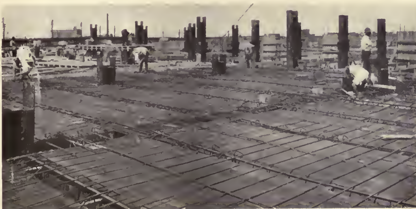
VIEW SHOWING SLAB REINFORCEMENT
